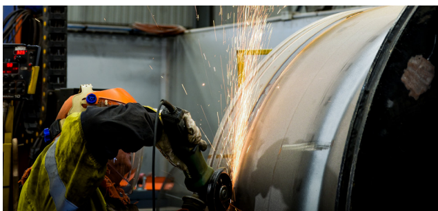
5. Machining (Repair Preparation)
