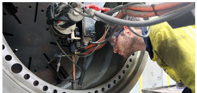
4. Welding (Section Replacement)
