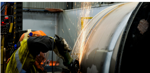
5. Machining (Repair Preparation)
