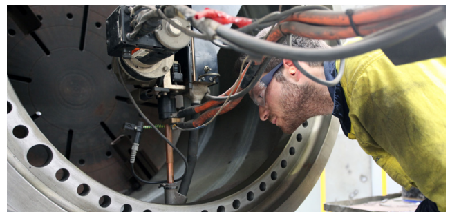
4. Welding (Section Replacement)
