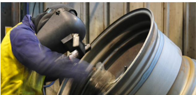
3. Welding (Section Replacement)
